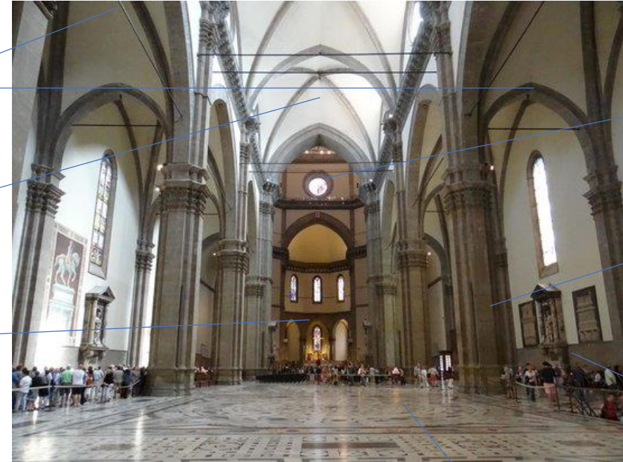
Pointed arch Groin gothic vault Apse
